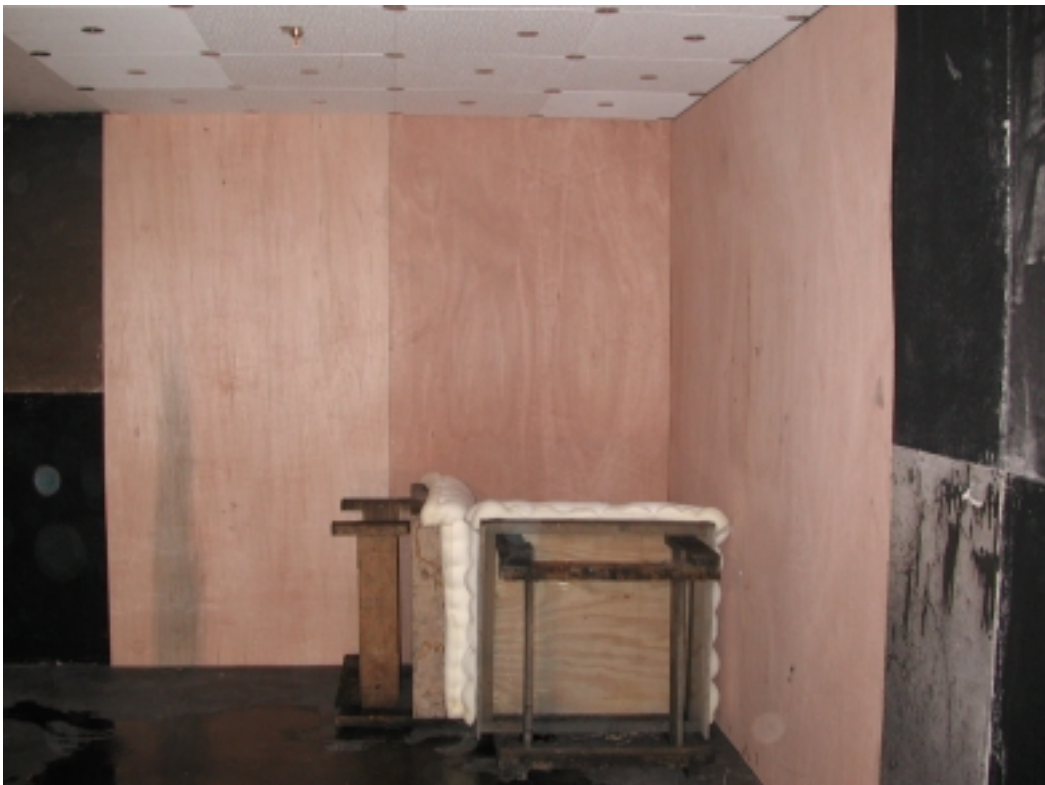
Figure A-4 The luxury cabin prior to the test. The photo shows the position of the nozzle closest to the corner.
