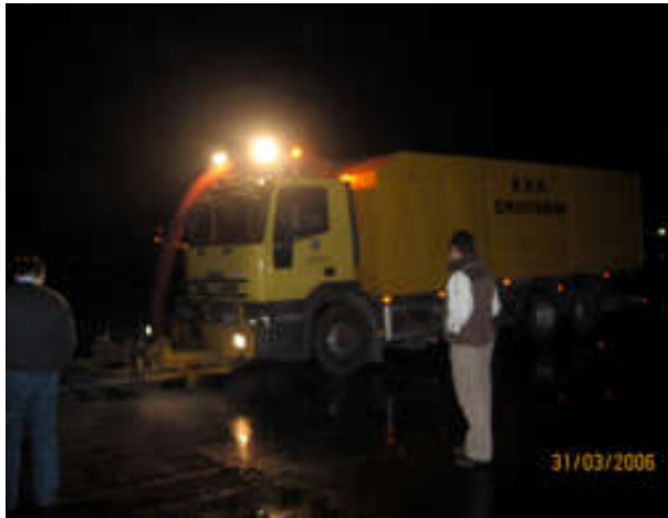
Picture 25 – 26 The tire track cleaning operation by compressed water jet
