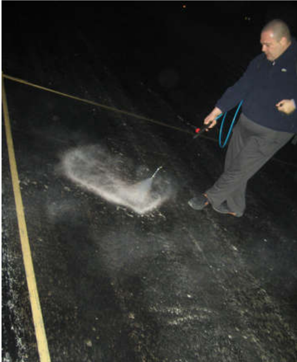
Picture 19 - Step 3 The application of neutralization solution 01:20
