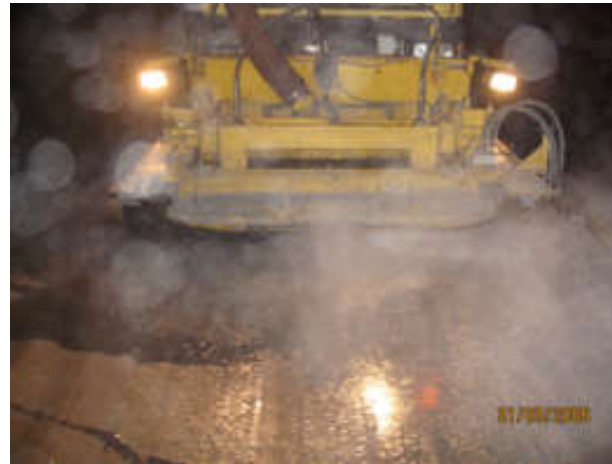
Picture 25 – 26 The tire track cleaning operation by compressed water jet
